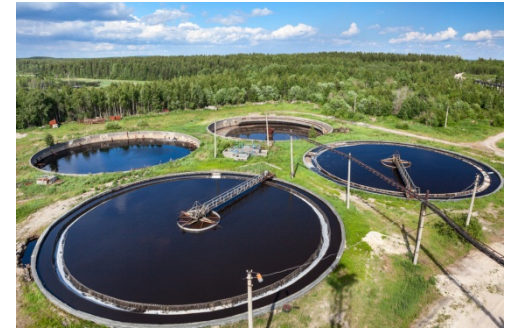
Coagulation and settling ponds
