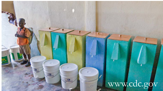
Slow sand filters in Haiti
